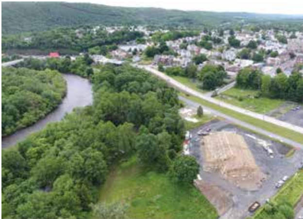
(Aerial picture of the Lehigh River and south side of town during the construction of the Lehighton Outdoor Center.)
